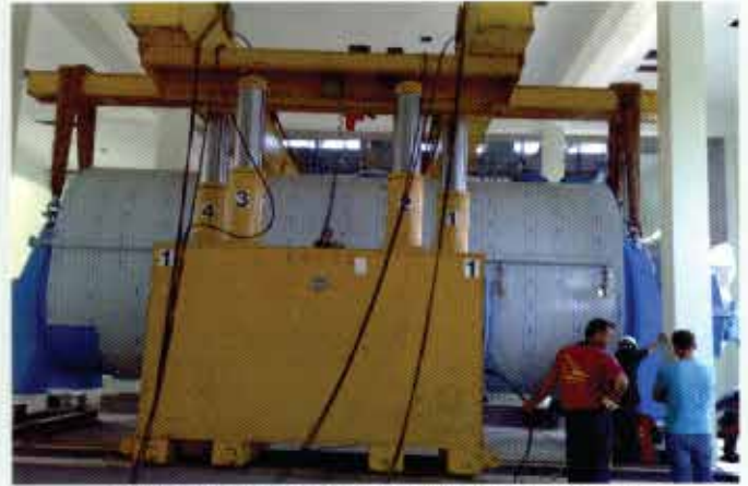
Installation of 6 pcs. of Sludge Dryers (70 tonnes each)
